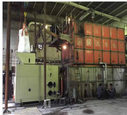
10 ton coal-fired boiler transformation
